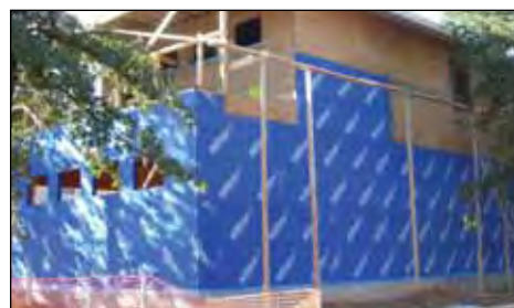
BlueskinVP provides a continuous plane of air-tightness to block the movement of air and moisture.
