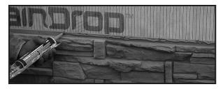
Apply no more than a ¼" bead of GenStone color matched caulking or polyurethane construction adhesive to all positive edges to ensure a watertight barrier. Smooth out the caulking bead with glove-protected finger, wiping away excess and leaving an even film of caulk so that panels have a snug fit. Remember, the positive shiplap edge should always be upright.
