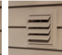
Louvered Exhaust Vent Louvered Exhaust Vent is used to vent dryers and bathroom exhaust fans.
